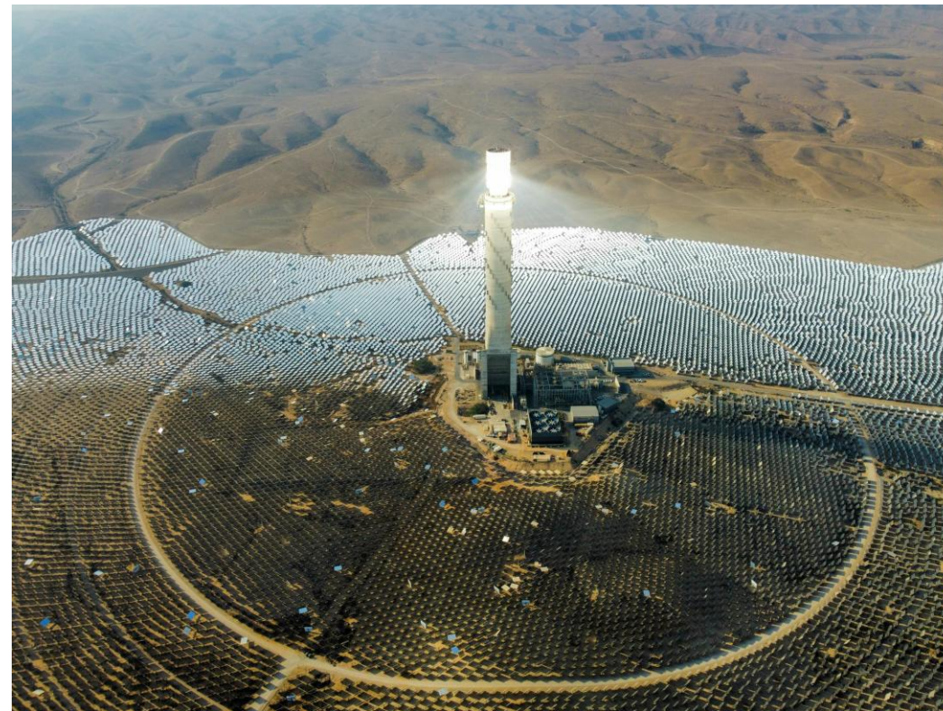
Concentrated Solar Power
